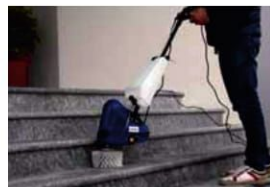
Cleaning of outside stairs
